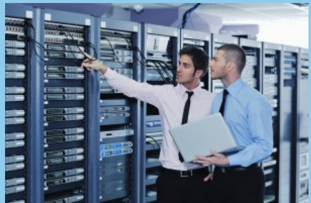
Audit IT Power Consumers and Assess Power Metering
