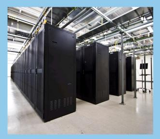
OpenData real-time monitoring allowed raising the chilled water temperature from 43°F to 52°F, which saved at least 15% of the chiller energy. The room temperature was also raised from 69°F to 74°F.
